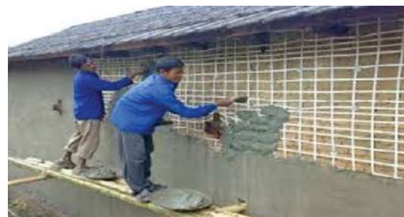
PP band for low strength masonry adobe structure
