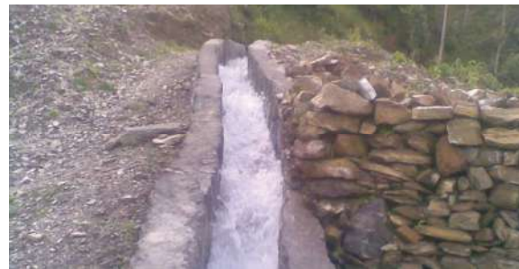
फोटो : Proper canal lining in hill, Kaski
