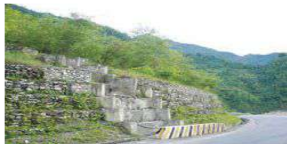
फोटो : Krishnavir Landslide before treatment
