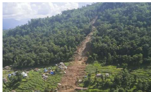
फोटो : Landslide in Parbat due to steep slope, soft slope material and intensive rainfall Source: Annapurna online news
