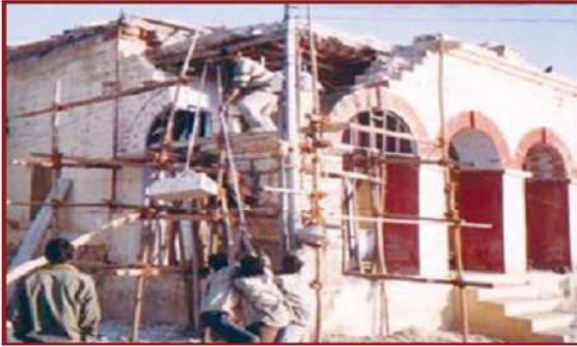
Cracked arcade being restored stone by stone
