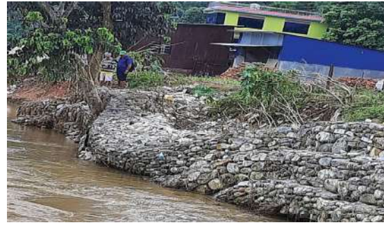
फोटो : Failure of Gabion Wall due to river bank scouring and poor construction method adopted, Damauli.
