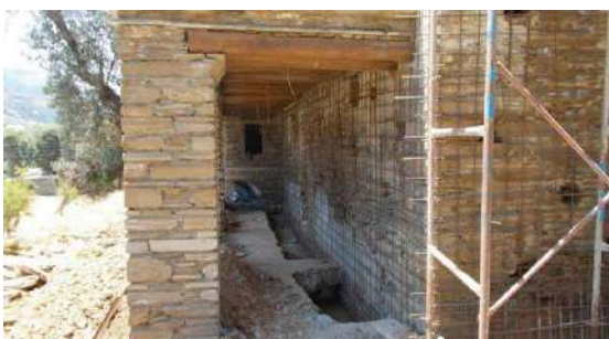
Jacking in Stone Masonry load bearing building
