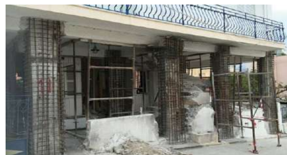
RC Jacketing in RCC frame system
