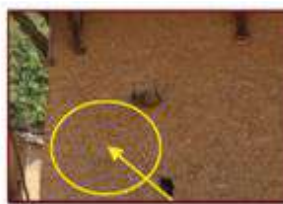
Wall having Grade 1 crack
