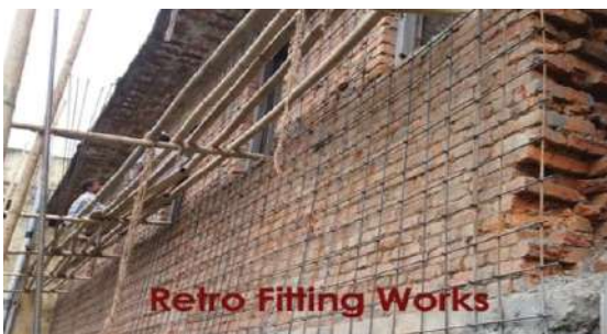
Jacketing Retrofitting in brick masonry load bearing building
