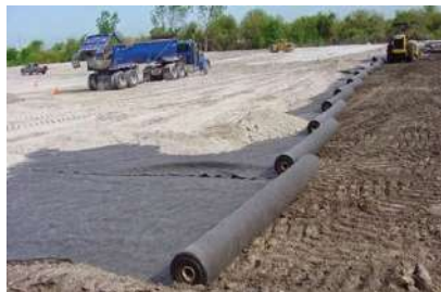
फोटो : Subgrade protection using geotextile
