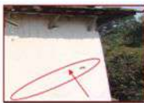
Wall having Grade 1 crack
