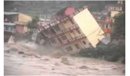
फोटो : Building swept away by Flood
