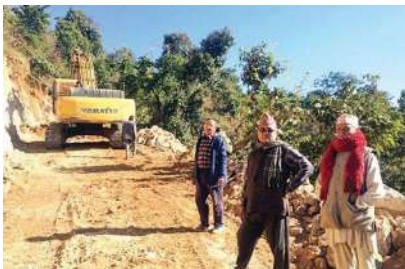
फोटो : Rural Road Construction
